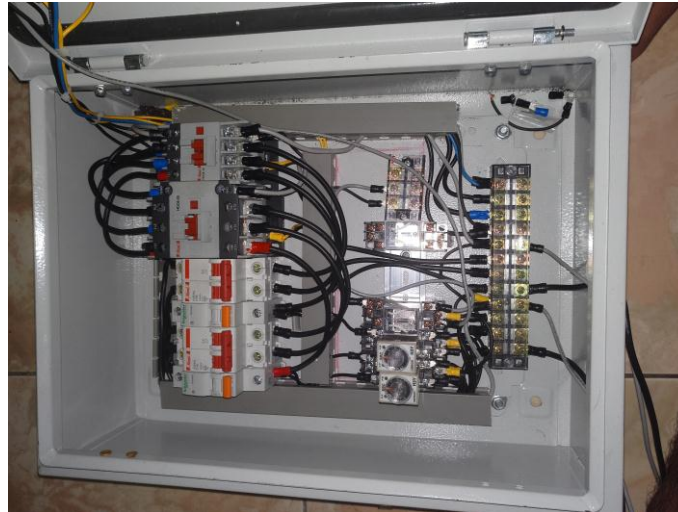
Gambar 2. Rangkaian Automatic Changeover Switch
